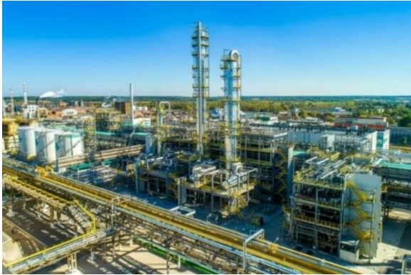
A modern ammonia production plant
