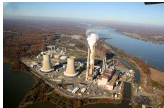
The Chalk Point Power Generating Plant located on the Patuxent River
